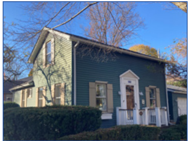
A one-and-a-half-story Folk house reminiscent of the I-house from the mid-nineteenth century. City of Birmingham, photo by KDG, 2022.
