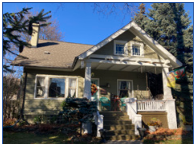
A Craftsman Bungalow with a gabled porch with battered wood piers resting on brick piers, rafter tails, and decorative windows in the gable end. City of Birmingham, photo by KDG, 2022.
