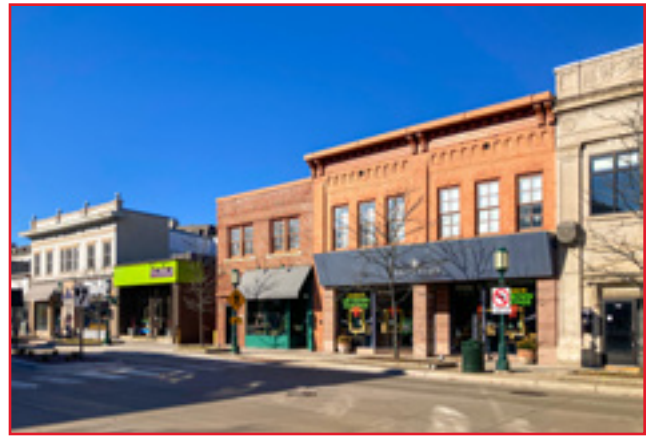
Rooftop mechanical equipment and penthouses that are present on these buildings within Birmingham's Commercial Historic District are positioned such that they are not visible from the public-right-of-way. Positioning rooftop mechanical equipment and penthouses in this manner is recommended. City of Birmingham, photo by KDG, 2022.
