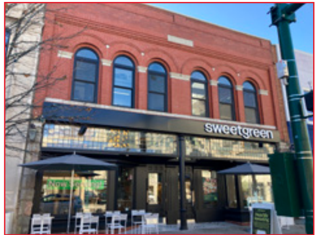
A typical historic storefront in the Central Business Historic District, with recessed entrances and large glass windows, City of Birmingham, photo by KDG, 2022.
