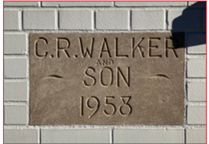
It is recommended that historic signage be retained. City of Birmingham, photo by KDG, 2022.
