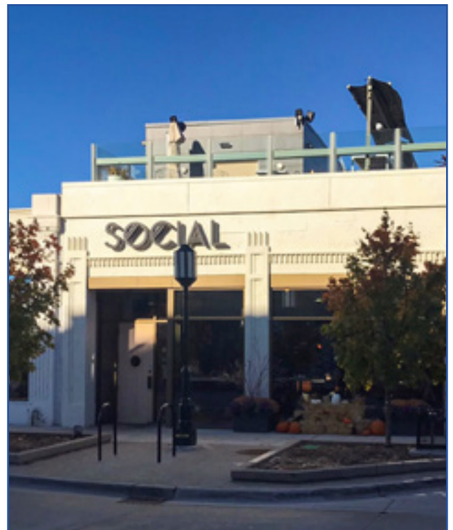
Small Art Deco building with geometric motifs paired with a smooth wall surface. City of Birmingham, photo by KDG, 2022.
