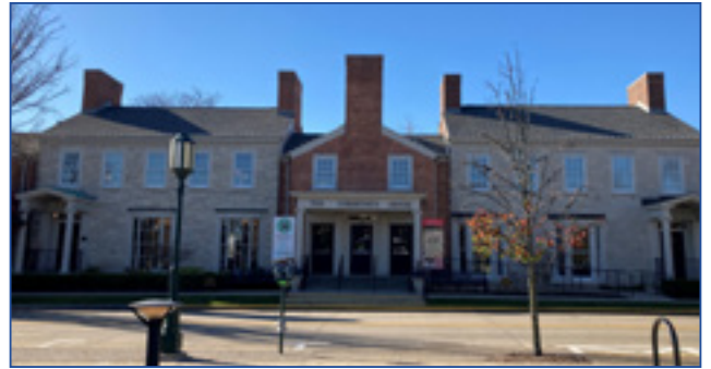
Birmingham's Community House exemplifies the Colonial Revival style with its classically inspired portico and entrance, denticulated cornice, 8-over-8 windows, and incorporation of large bay windows not usually found in original colonial buildings. Portions of this building are contemporary additions constructed in the Colonial Revival style to match the historic core building. City of Birmingham, photo by KDG, 2022.
