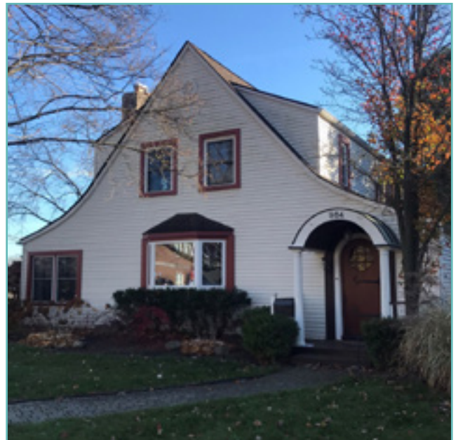
The replacement of historic windows with a modern, vinyl bay window with no muntins is not recommended as it does not match the historic window. City of Birmingham, photo by KDG, 2022.
