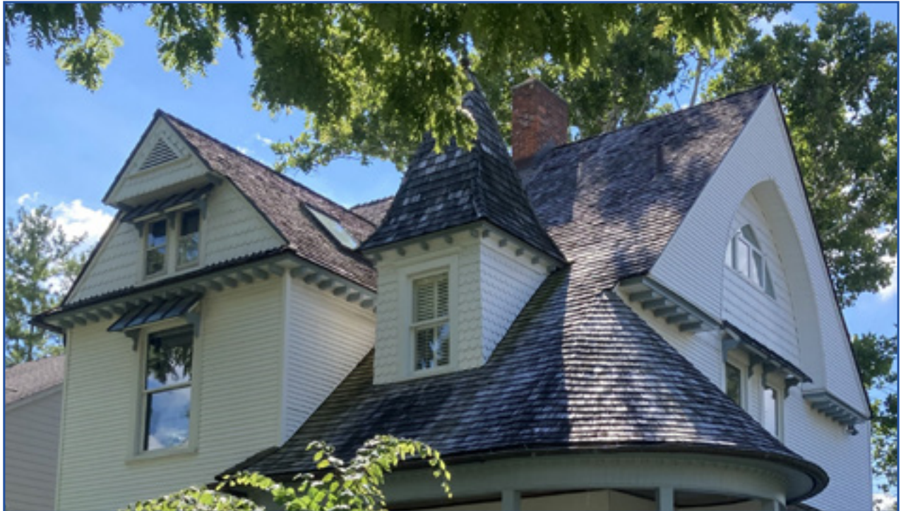
Multiple roof shapes are characteristic of the Queen Anne style. City of Birmingham, photo by KDG, 2022.
