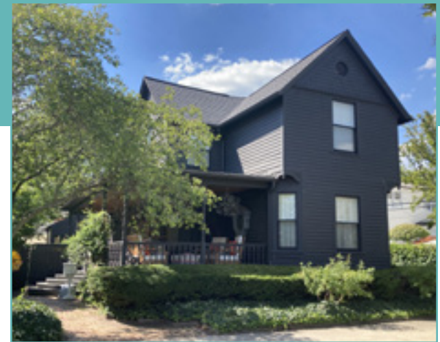
This exterior elements of this Folk Victorian home are well maintained. City of Birmingham, photo by KDG, 2022.
