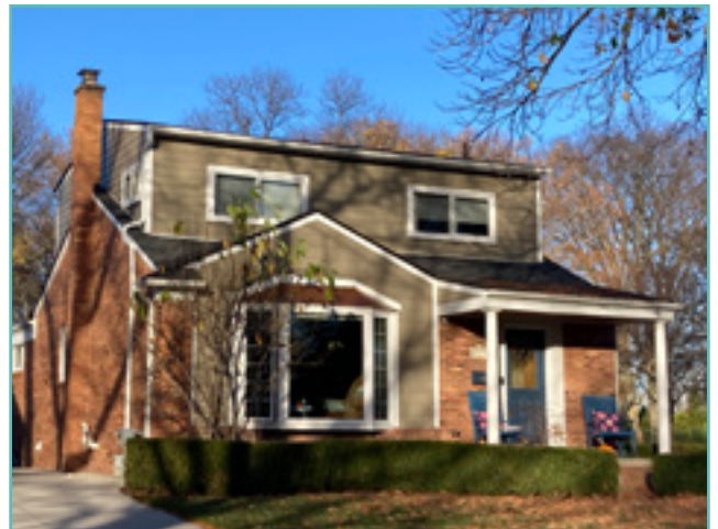
This second-story addition would not be recommended as it is highly visible. City of Birmingham, photo by KDG, 2022.
