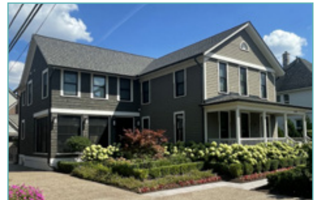
The placement of this addition to the left of the historic home is acceptable as it does not overwhelm this historic portion of the home and is placed near the rear. Bates Street Historic District, City of Birmingham, photo by KDG, 2022.
