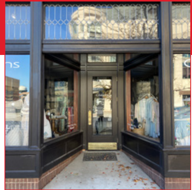
Preservation of historic storefront elements such as the recessed entry and leaded glass transoms is recommended. Central Business Historic District, City of Birmingham, photo by KDG, 2022.
