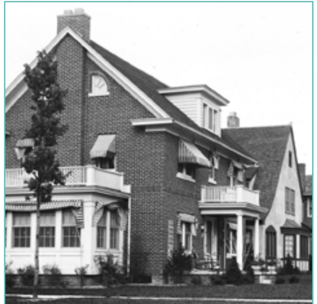
Historic residential awnings are illustrated in the above image. Triangular, striped fabric awnings with scalloped edges were commonly used on residences. Image is used courtesy of the Walter P. Reuther Library, Archives of Labor and Urban Affairs, Wayne State University. City of Birmingham, photo by KDG, 2022.
