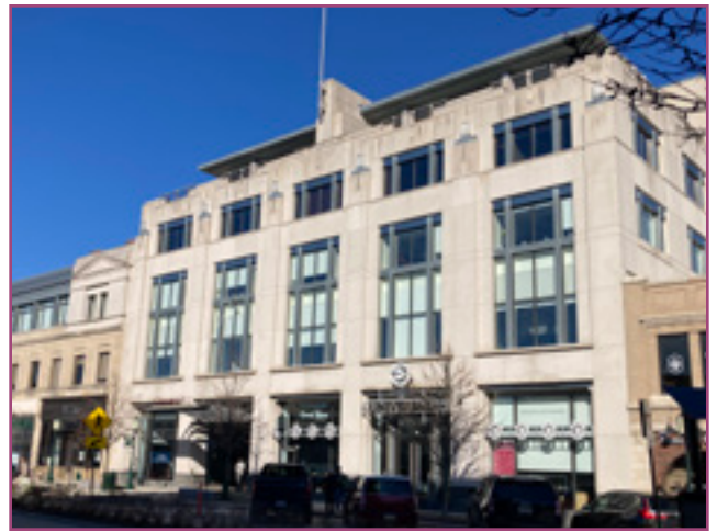
The scale and massing of this newer, non-historic building significantly differs in size from the surrounding Central Business District Historic District as it is both taller than any of the historic structures and much larger. The historic buildings in the Central Business District are primarily comprised of two and three story buildings. City of Birmingham, photo by KDG, 2022.
