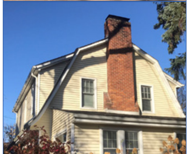
The gambrel roof with flared eaves paired with a large, shed roof dormer are characteristic of the Dutch Colonial Revival style. City of Birmingham, photo by KDG, 2022.
