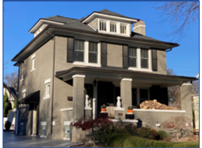
The Prairie style, with the characteristic hipped roof, hipped roof dormers, widely overhanging eaves, and large porch, is often applied to the American Foursquare form. City of Birmingham, photo by KDG, 2022.
