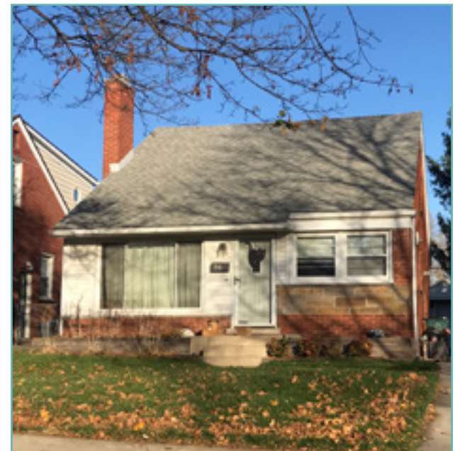
Modest, mid-twentieth century homes are worthy of preservation and should not be overlooked. City of Birmingham, photo by KDG, 2022.
