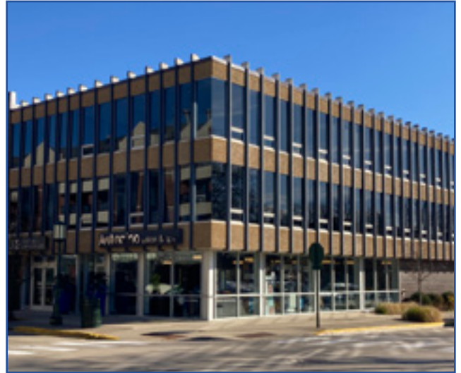
Modern buildings often incorporate new materials, with the building above incorporating expanses of glass and pebbled spandrels into the design. City of Birmingham, photo by KDG, 2022.
