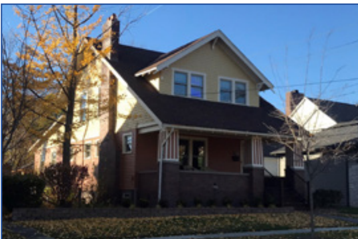
A large Craftsman Bungalow with a front gable dormer, full-width porch with brick piers topped with battered wood piers, and extended eaves with rafter tails and knee brackets. City of Birmingham, photo by KDG, 2022.
