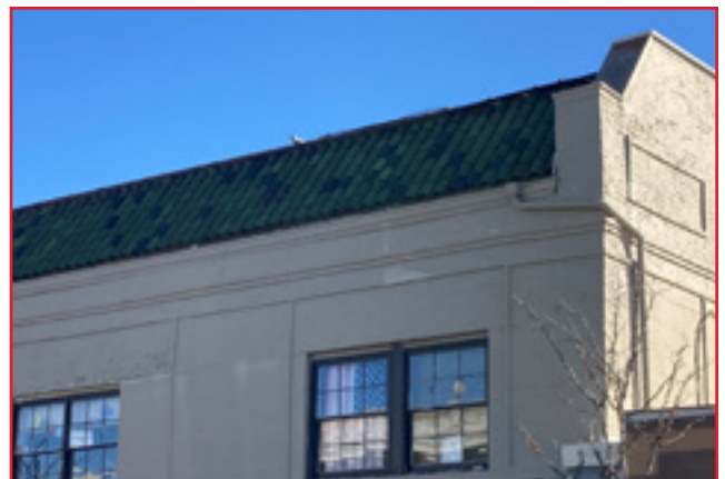
Clay tile roof in the Central Business Historic District, City of Birmingham, photo by KDG, 2022.
