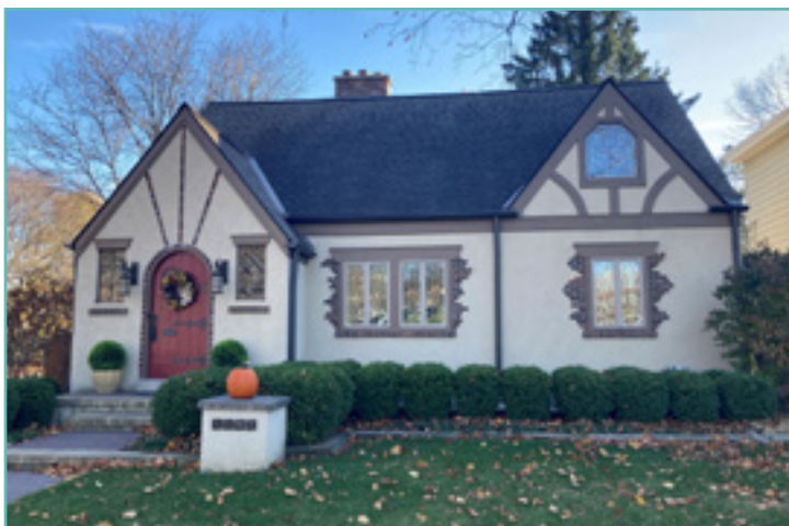
The storm windows above are not recommended as their color does not match the window sashes. City of Birmingham, photo by KDG, 2022.
