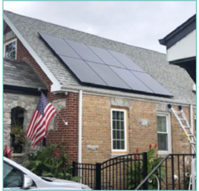
Solar panels placed in an acceptable location on the secondary plane of a side gabled roof, Google Image, 2022.
