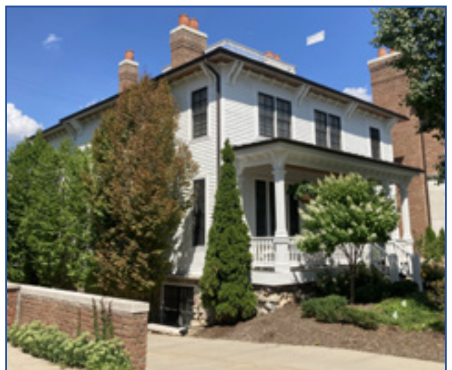
The Schuyler House in the Merrill-Townsend-Brown Neighborhood is an Italianate style house with over hanging eaves, brackets, and tall, narrow windows. City of Birmingham, photo by KDG, 2022.
