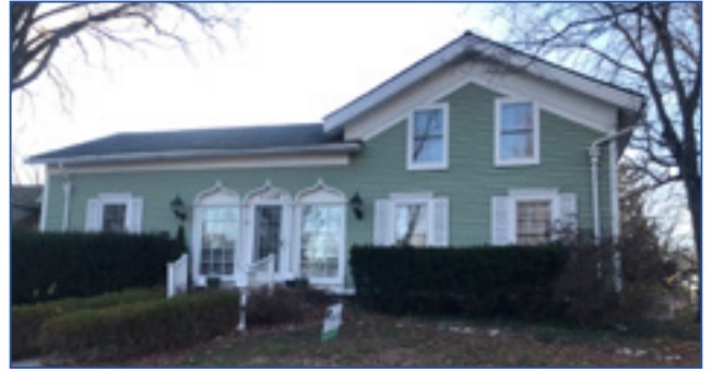
The Daniels House is an example of the Greek Revival style with its prominent entablature, 6-over-6 windows, and shallow gable roof. The ogee arches near the center of the building would have once been open, accessing a loggia. The Upright and Wing form is characteristic of Folk architecture in southeastern Michigan. City of Birmingham, photo by KDG, 2022.
