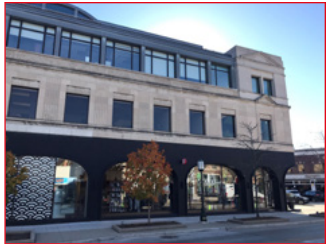
Large and prominent additions that are visible on the primary façades are not recommended, City of Birmingham, photo by KDG, 2022.
