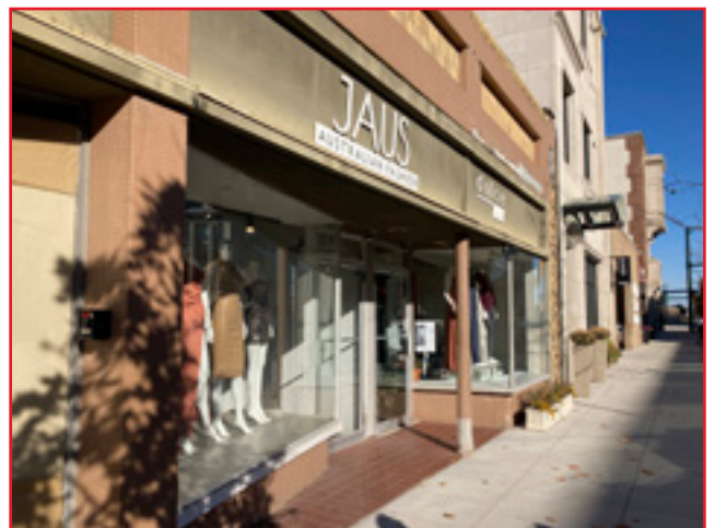
A mid-century storefront in the Central Business Historic District likely replaced an earlier storefront design. The new storefront utilizes large expanses of glass and a recessed entrance. City of Birmingham, photo by KDG, 2022.
