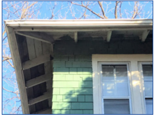
Exposed, extended eaves with visible rafters are characteristics of the Craftsman style. City of Birmingham, photo by KDG, 2022.
