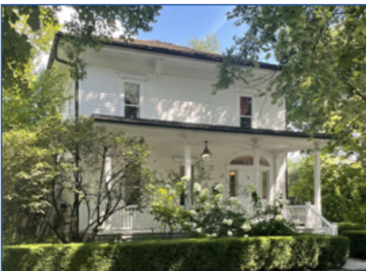
The John W. Perry House in the Bates Street Historic District is an Italianate style house with over hanging eaves, brackets, and tall, narrow windows. City of Birmingham, photo by KDG, 2022.
