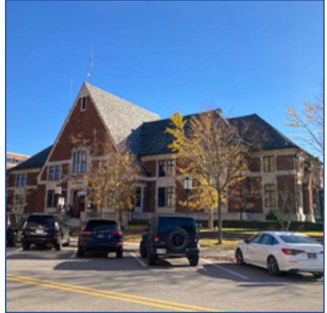
City Hall, Shain Park Historic District, City of Birmingham, photo by KDG, 2022.
