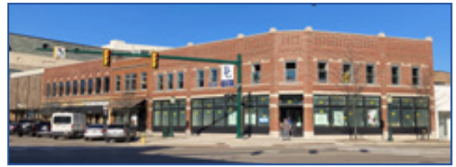
Parks Building, Central Business Historic District, City of Birmingham, photo by KDG, 2022.
