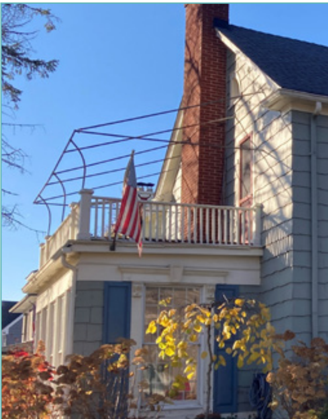
It is recommended that historic rooftop balconies be preserved. City of Birmingham, photo by KDG, 2022.
