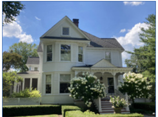
The hipped roof with lower cross gables, mixture of wood shingles and weatherboard, large porch, bay window, and irregular shape are characteristic of the Queen Anne style. City of Birmingham, photo by KDG, 2022.
