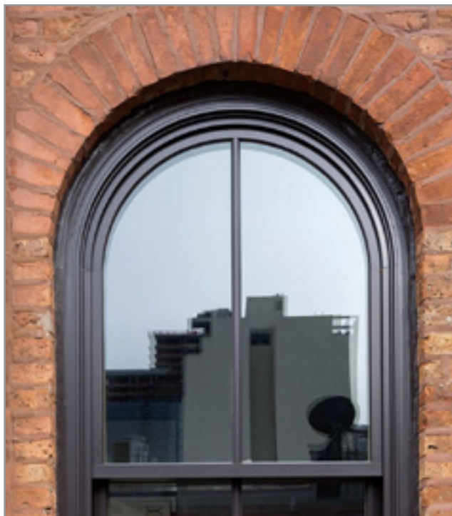
If repair or replacement of historic windows is not feasible, aluminum clad windows provide a potential solution that are capable of achieving the profile, depth, and colors of historic windows. Photo courtesy of AVI Windows and Doors.
