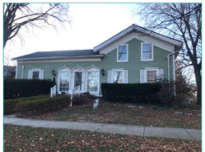
The enclosure of the historic, ogee arch loggia on this Greek Revival house occurred long ago and may now be considered part of the historic character of the house.
