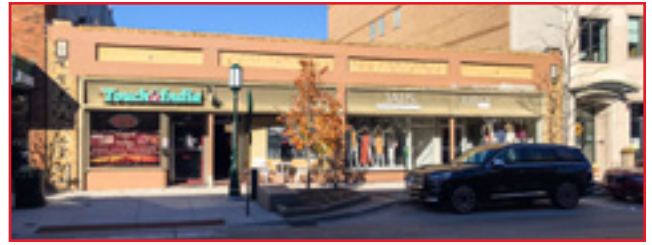
Commercial buildings typically have flat roofs that are obscured by masonry parapets, shielding the roof from view. City of Birmingham, photo by KDG, 2022.
