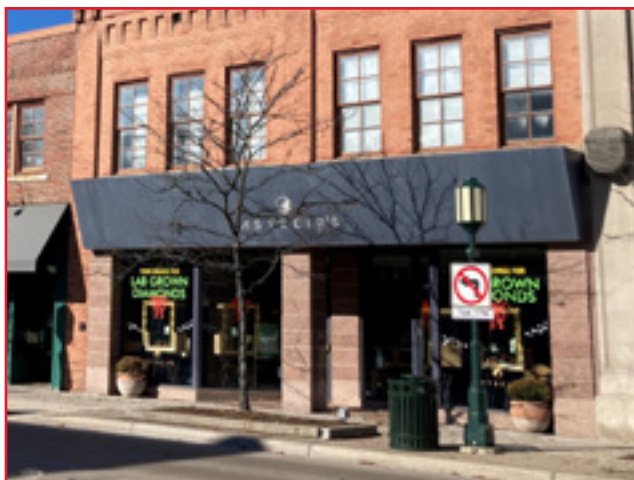
The modern awning here is an inverted version of the historic awning and is not recommended for use on historic buildings. City of Birmingham, photo by KDG, 2022.
