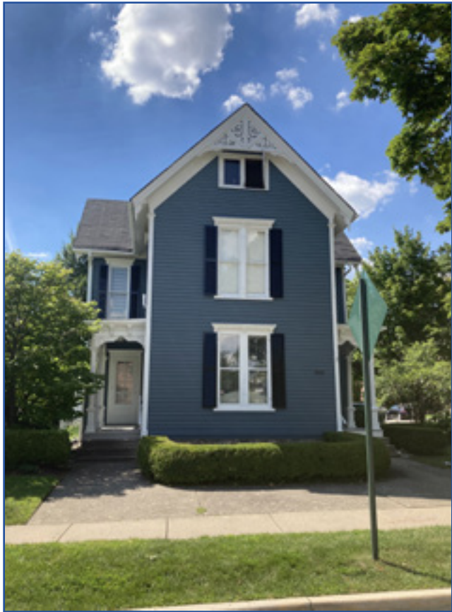
The presence of frieze work, gable decoration, tall and narrow rectangular windows, and decorative window cornices indicate the Folk Victorian style. City of Birmingham, photo by KDG, 2022.
