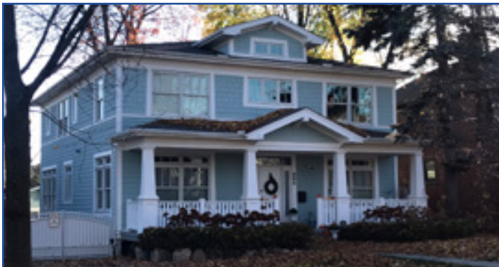
Battered wood piers, a large full-width porch, 3-over-1 windows, and protruding roof beams are some of the Craftsman details applied to this large Foursquare form. City of Birmingham, photo by KDG, 2022.
