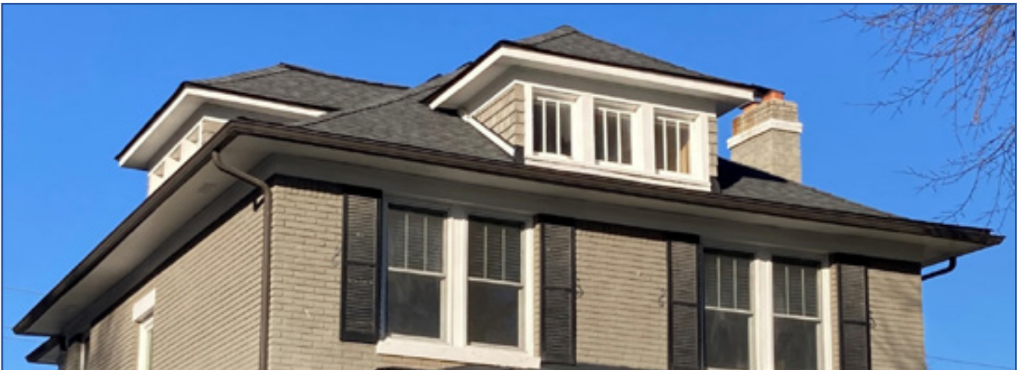
Closeup image of the hipped roof, hipped roof dormers, widely overhanging eaves, and 3-over-1 windows. City of Birmingham, photo by KDG, 2022.
