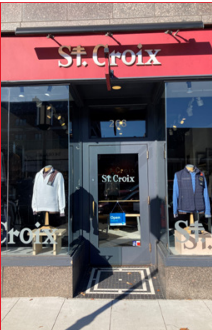
Typical storefront in the Central Business Historic District, City of Birmingham, photo by KDG, 2022.
