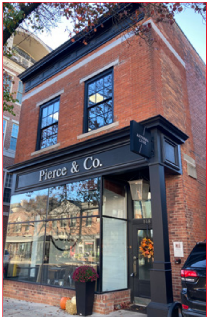
Typical storefront in the Central Business Historic District, City of Birmingham, photo by KDG, 2022.
