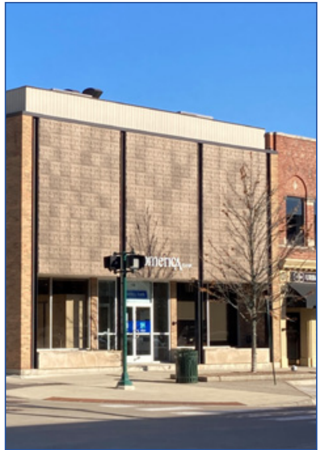
Verticality is emphasized by the narrow windows and solid spandrels organized in columns on the side elevation. The use of molded, textured panels on the façade is also characteristic of Modern buildings. City of Birmingham, photo by KDG, 2022.
