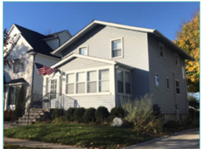
Enclosing porches for additional living space is particularly common on modest dwellings.
