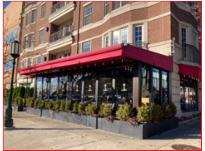
Patios such as this with a historically sensitive awning, use of finished materials, and appropriate scale are recommended, City of Birmingham, photo by KDG, 2022.
