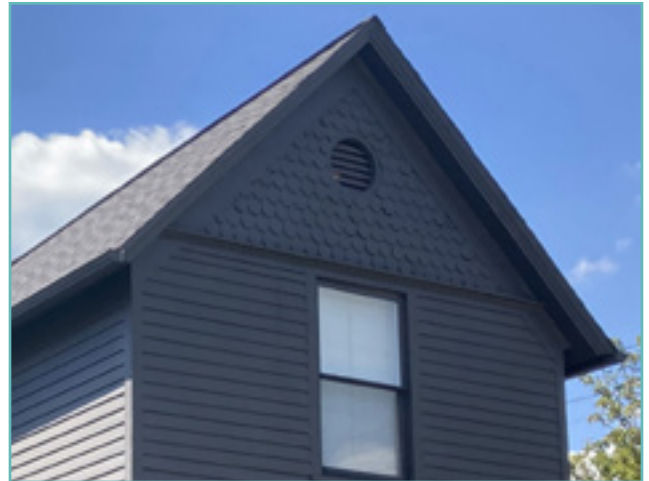
Narrow, historic wood siding and historic wood shingles. City of Birmingham, photo by KDG, 2022.
