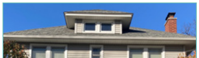
Hipped roof dormers are character defining elements of Craftsman style and Prairie style houses. City of Birmingham, photo by KDG, 2022.
