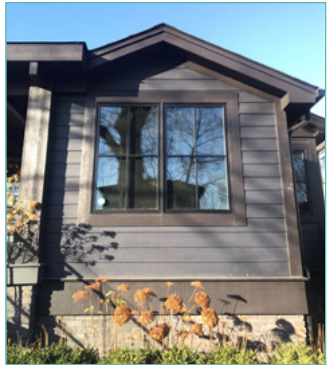
Although this modern replacement siding has a different finish than historic wood siding, the texture and dimensions make it a viable replacement for wood cladding too deteriorated to repair or preserve. City of Birmingham, photo by KDG, 2022.
