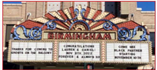
The preservation of exterior theatre lighting displays is recommended, City of Birmingham, photo by KDG, 2022.
