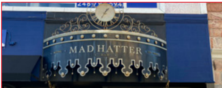
Canopies of unique design are acceptable on historic commercial buildings as long as they respect the scale and size of nearby canopies and do not harm historic materials or obscure historic building details. City of Birmingham, photo by KDG, 2022.
