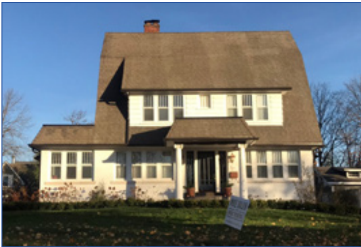
A large gambrel roof with a shed roof dormer. The facades of Dutch Colonial Revival houses are often symmetrical. City of Birmingham, photo by KDG, 2022.
