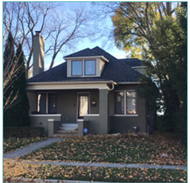
If circumstances require that modern window replacements are used, it is recommended that replacement windows match the historic windows as closely as possible. The replacement windows shown above would not be recommended as they are fixed sash windows without muntins, which do not match the historic 3-over-1 windows that were originally present. City of Birmingham, photo by KDG, 2022.
