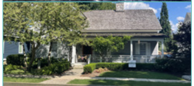
The maintenance, repair, and preservation of wood shingle roofs is recommended. City of Birmingham, photo by KDG, 2022.
