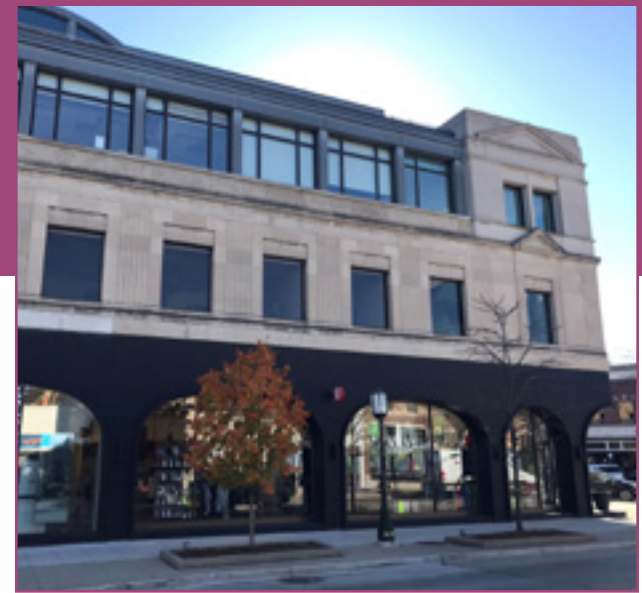
Large and prominent additions that are visible on the primary facades are not recommended, City of Birmingham, photo by KDG, 2022.
