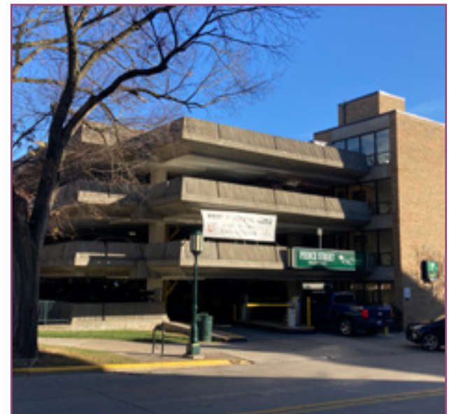
The Pierce Street Garage is a Brutalist style parking structure that, while not located in a historic district, is directly adjacent to the Shain Park Historic District. While the scale of the garage is compatible with the district, it does not incorporate street level commercial space which is a recommendation for newly built parking garages. City of Birmingham, photo by KDG, 2022.
