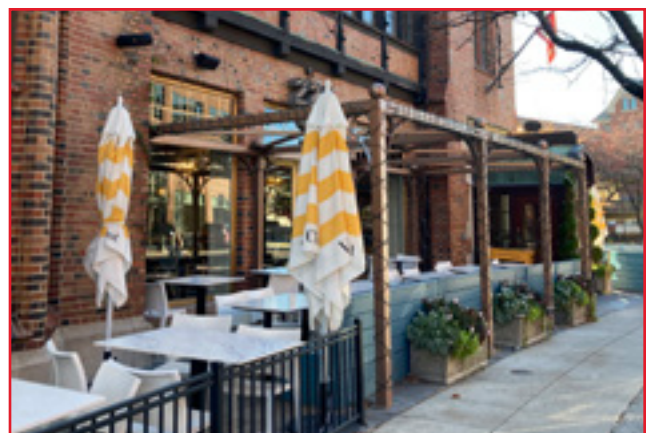
Cafe patio construction that is fastened/mounted to the building is not recommended. City of Birmingham, photo by KDG, 2022.
