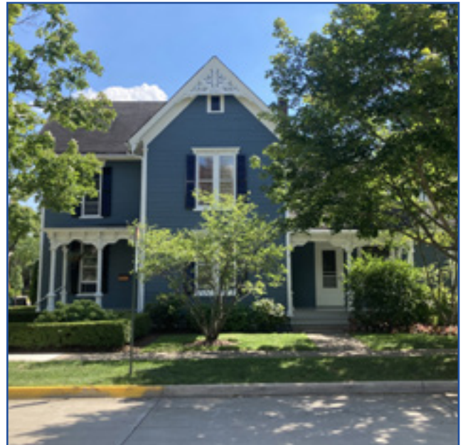
Langley House, Merrill-Townsend-Brown Neighborhood, City of Birmingham, photo by KDG, 2022.
