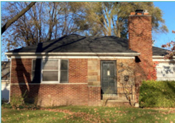
Use of brick veneer and stone veneer on a small Ranch house. City of Birmingham, photo by KDG, 2022.
