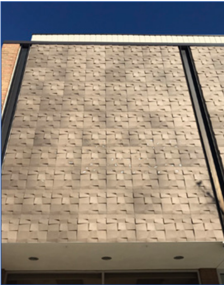
View of textured panels. City of Birmingham, photo by KDG, 2022.
