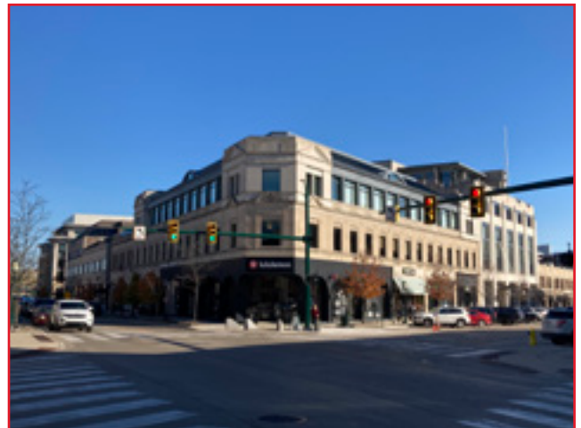
Large and prominent additions that are visible on the primary façades are not recommended, City of Birmingham, photo by KDG, 2022.
