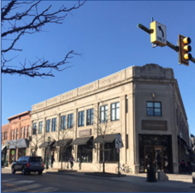
Ford Building, Central Business Historic District, City of Birmingham, photo by KDG, 2022.
