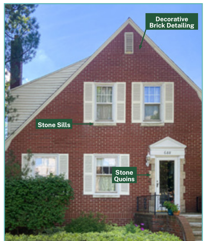
Brick and stone are common exterior wall materials in Birmingham. City of Birmingham, photo by KDG, 2022.
