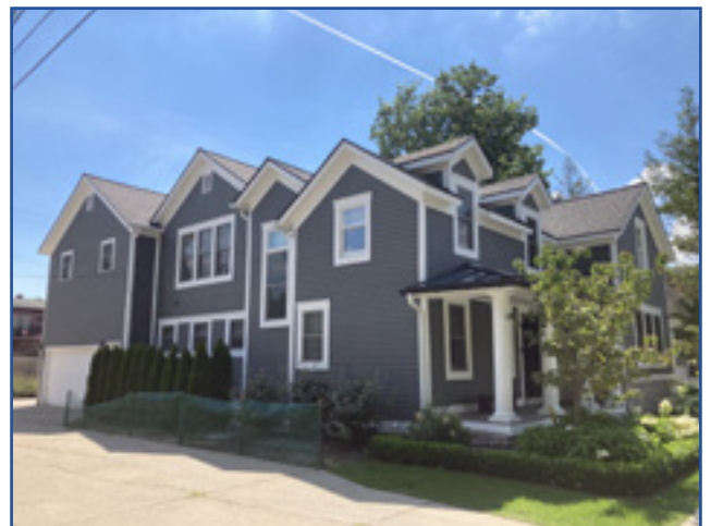
The original portion of this house is an Upright and Wing. City of Birmingham, photo by KDG, 2022.
