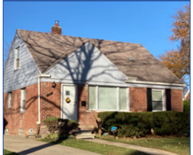
These examples illustrate the small front-facing gable often found on Minimal Traditional houses. City of Birmingham, photo by KDG, 2022.
