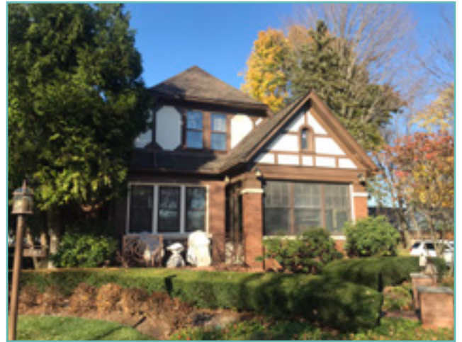
The screened and glazed porch of this Tudor Revival style house may have originally been open. City of Birmingham, photo by KDG, 2022.
