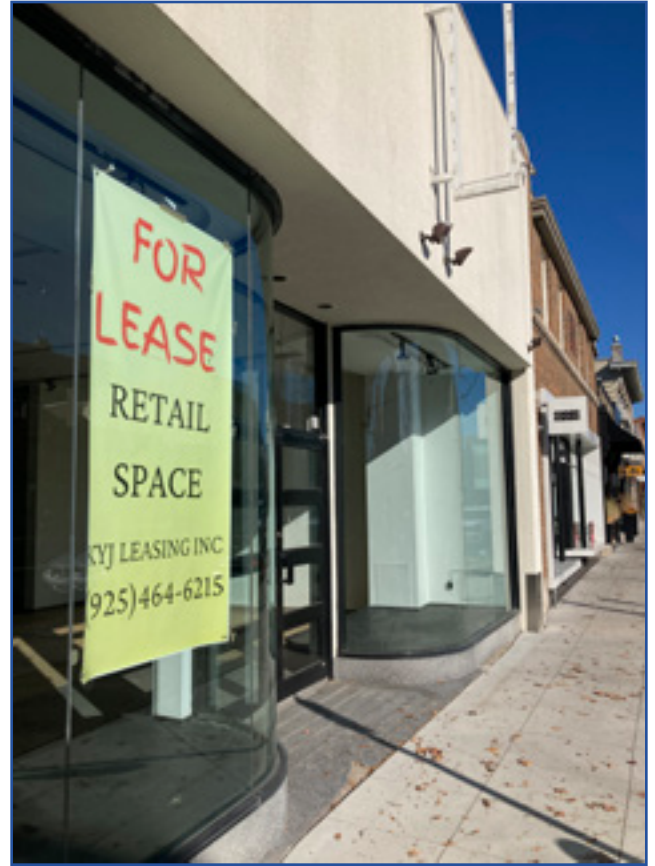
The curved corners with curved glass and stark façade are indicative of Streamline Moderne. City of Birmingham, photo by KDG, 2022.
