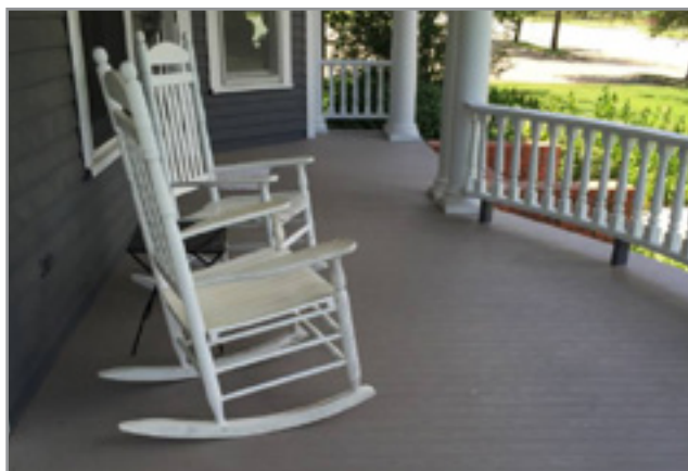
Selecting historically appropriate colors, dimensions, and textures can make the use of composite decking a viable alternative if repair or replacement of a historic wood porch or patio is not possible. Photo courtesy of Buck the Builder.
