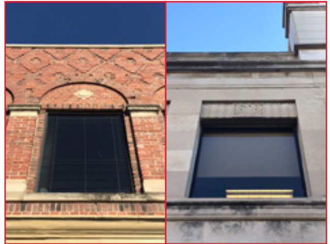
The replacement of historic windows with modern, fixed-sash windows is not recommended as it alters historic, character defining features of the building. Central Business Historic District, City of Birmingham, photo by KDG, 2022.
