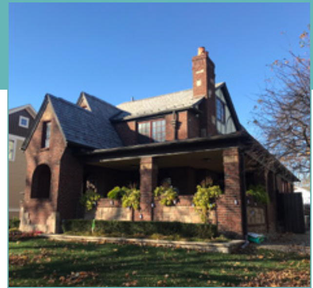
Porches were common components of historic residences and should be preserved. City of Birmingham, photo by KDG, 2022.
