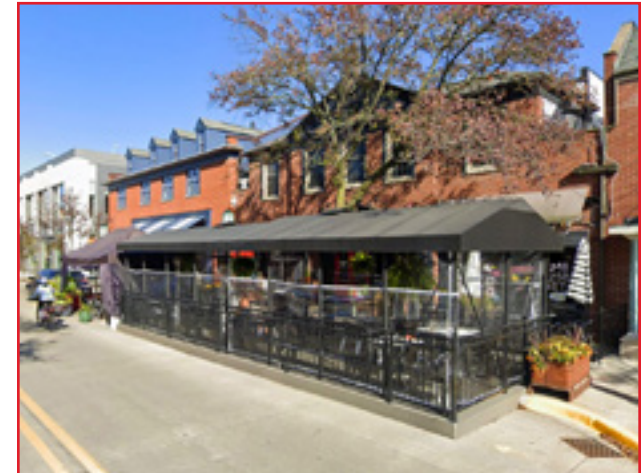
Sidewalk patio construction should be freestanding and not mounted or mechanically fastened to the façade, as shown here. Central Business Historic District, City of Birmingham, photo by KDG, 2022.
