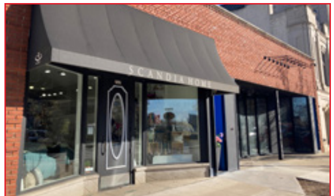
The replacement door above is not complementary to the historic building's style, and is therefore not recommended. Central Business Historic District, City of Birmingham, photo by KDG, 2022.
