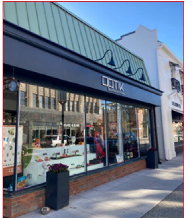
Metal trim is a common exterior cladding material. City of Birmingham, photo by KDG, 2022.
