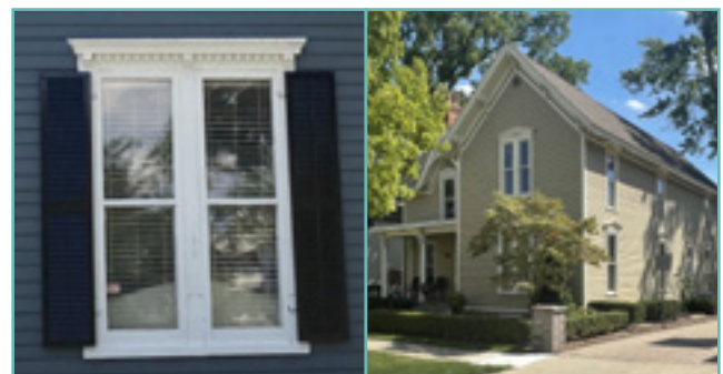
The maintenance, repair, and preservation of historic wood windows is recommended. Tall, narrow windows are character defining features of Victorian Period houses. City of Birmingham, photo by KDG, 2022.
