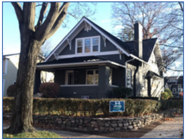
This Craftsman style house has knee brackets, a large porch with massive brick piers, a gabled roof, and 3-over-1 windows. City of Birmingham, photo by KDG, 2022.
